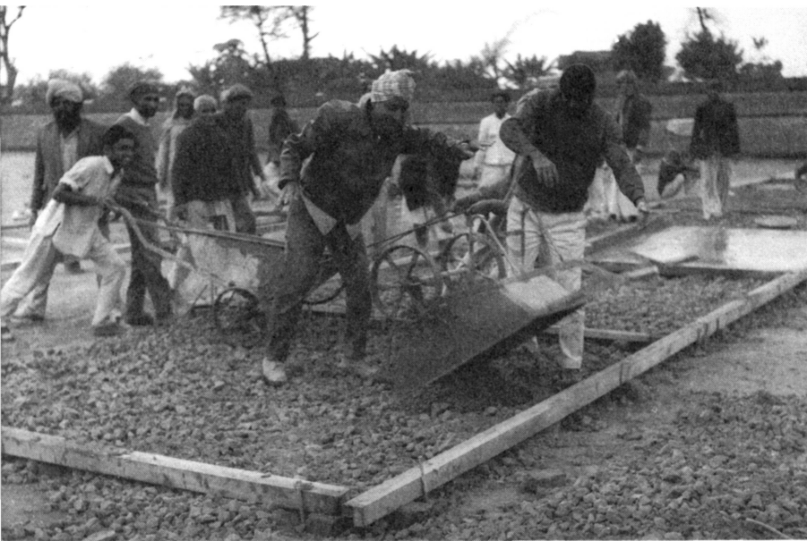
The huge quantities of concrete were prepared in a mixer and poured in sections.
